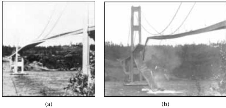
**Figure 13.23** (a) In 1940 turbulent winds set up torsional vibrations in the Tacoma Narrows Bridge, causing it to oscillate at a frequency near one of the natural frequencies of the bridge structure. (b) Once established, this resonance condition led to the bridge's collapse.
